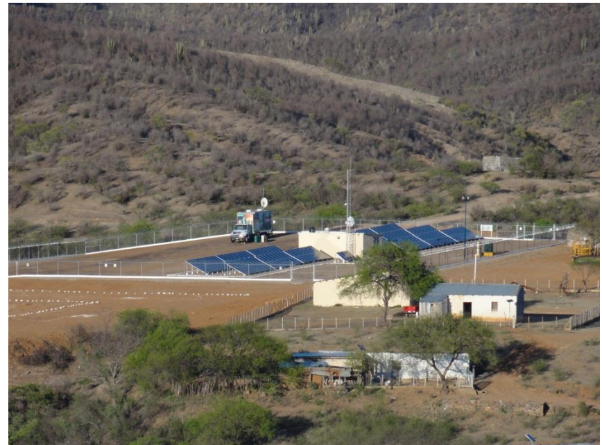
Hybrid PV Systems and Mini-Grids Fraunhofer ISE
