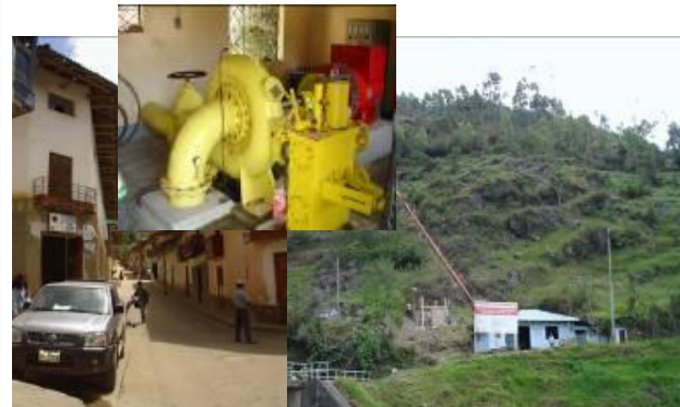
Hydroelectric power stations
