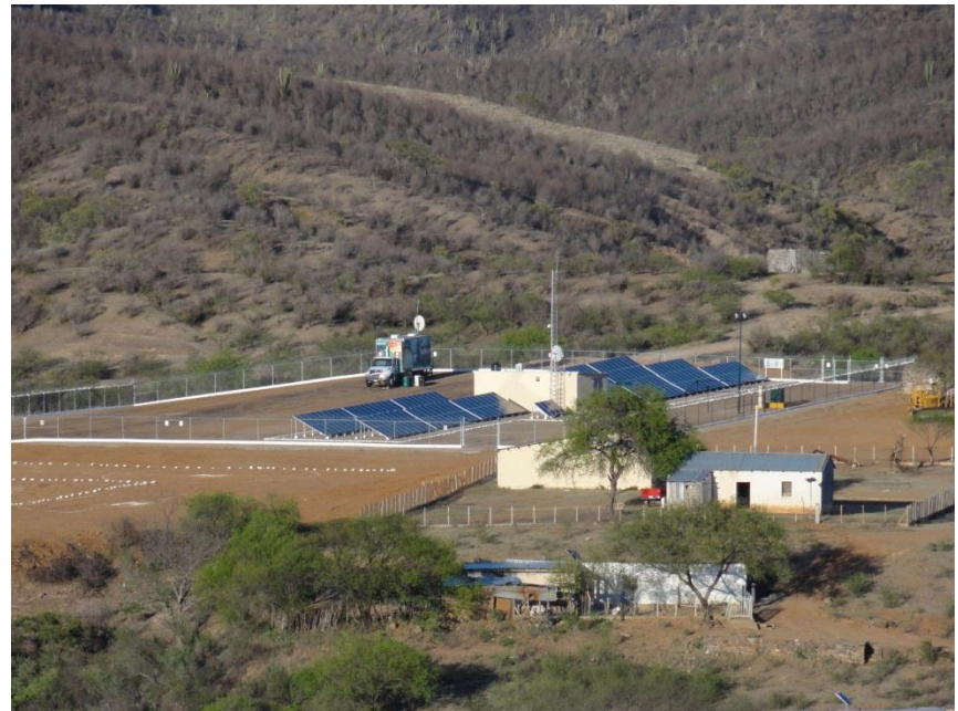
Hybrid PV Systems and Mini-Grids Fraunhofer ISE
