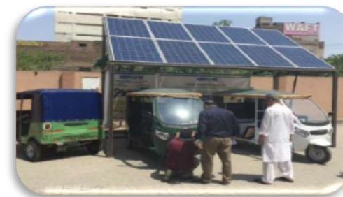
EV + Solar Fast Charging
