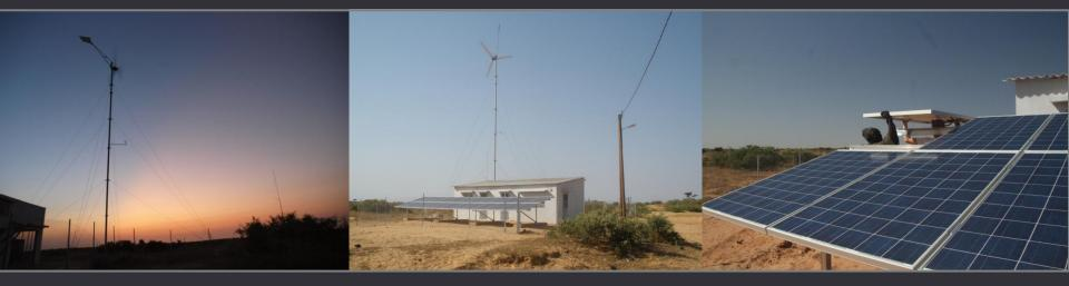
Foto: Wind-Solar-Diesel hybrid power system with battery storage for village power supply designed and operated by INENSUS West Africa
