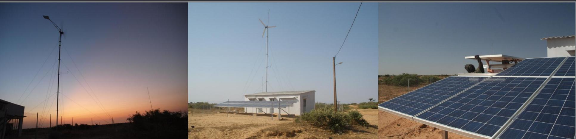
Foto: Wind-Solar-Diesel hybrid power system with battery storage for village power supply designed and operated by INENSUS West Africa
